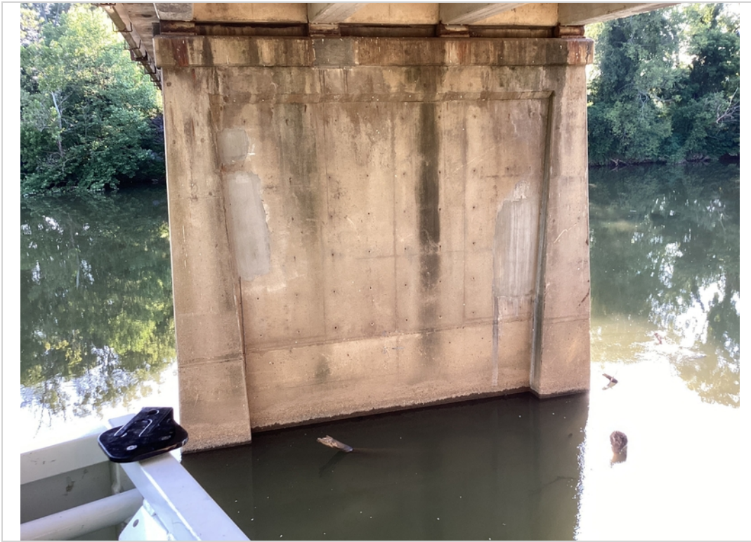
Spall repairs pier #2
