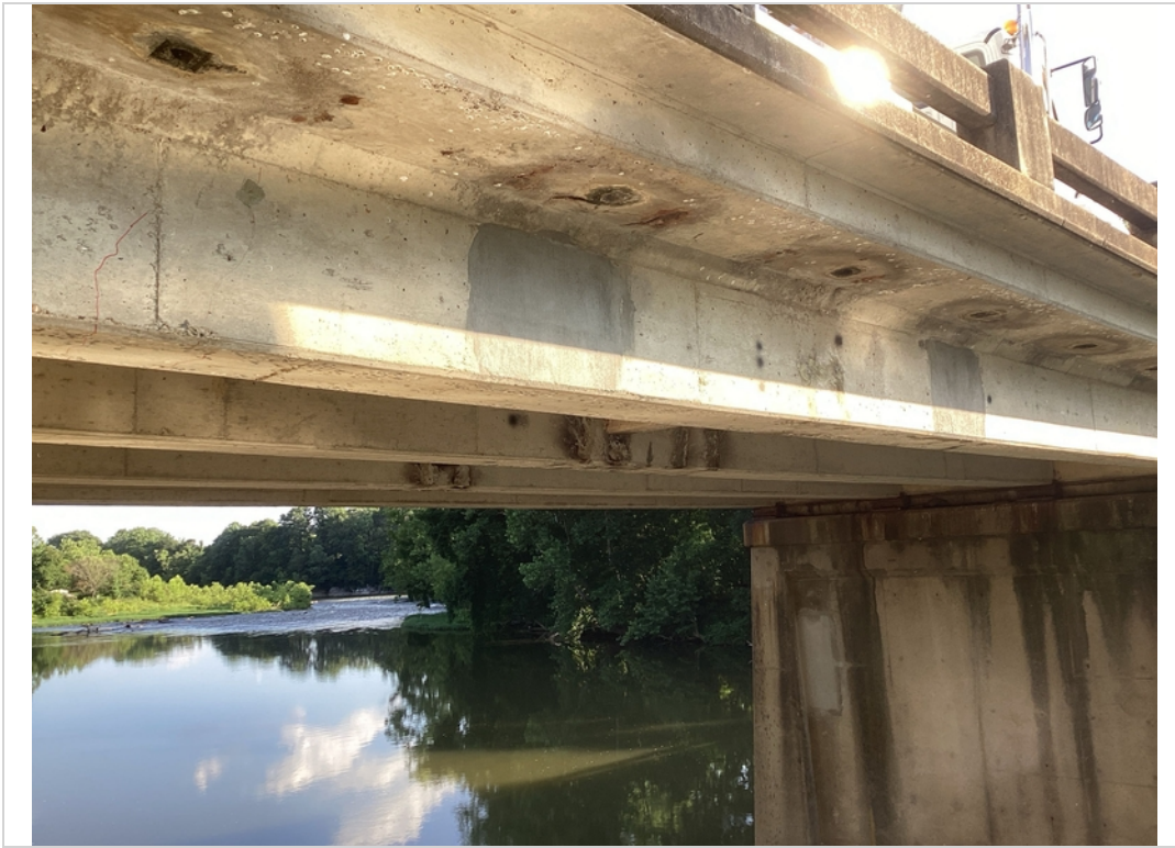
Patches on beam "D" span #4
