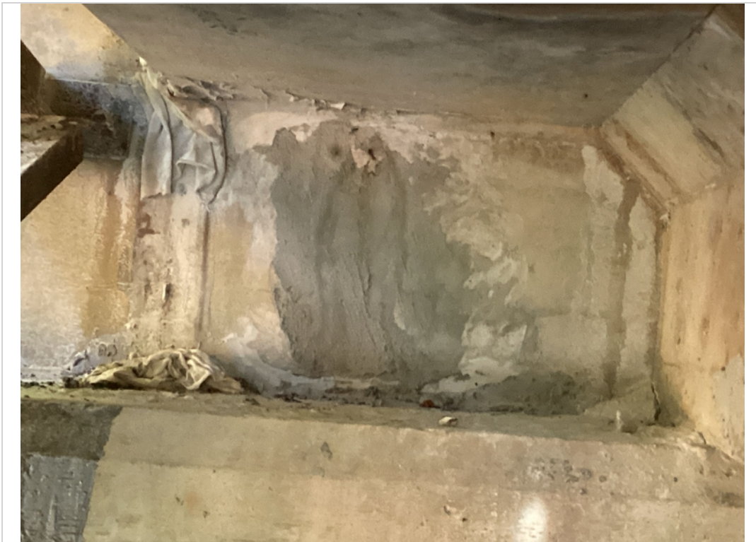
Previous cracks in abutment #2 backwall have been repaired
