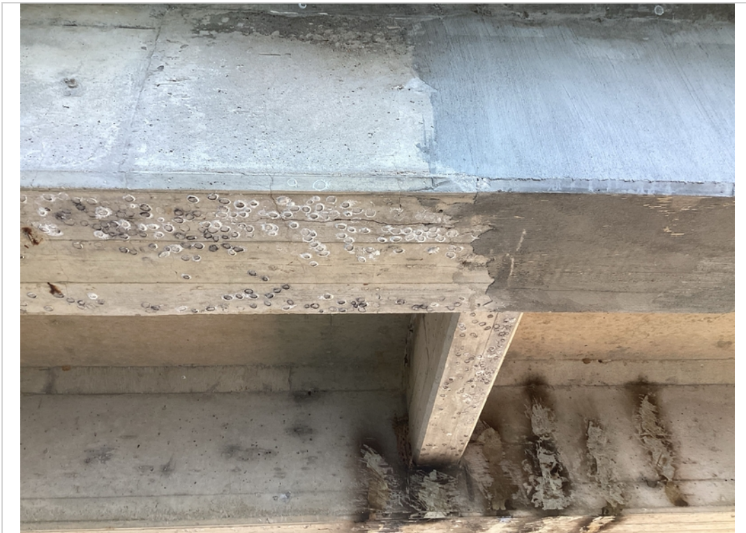
Hairline to 1/8" longitudinal crack beam "A" at midspan span #6
