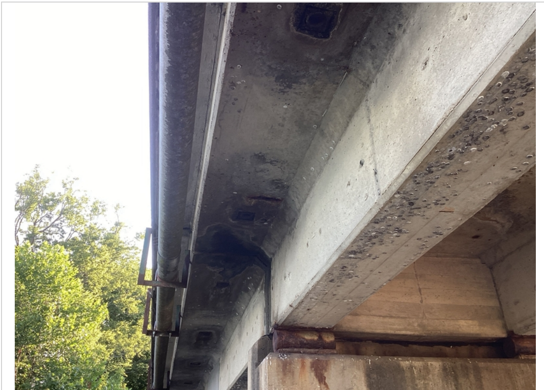
Span #5: In place spall/delamination and high steel popout span #5 left overhang
