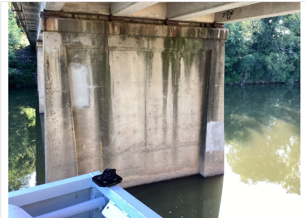
Spall and delamination repairs pier #3
