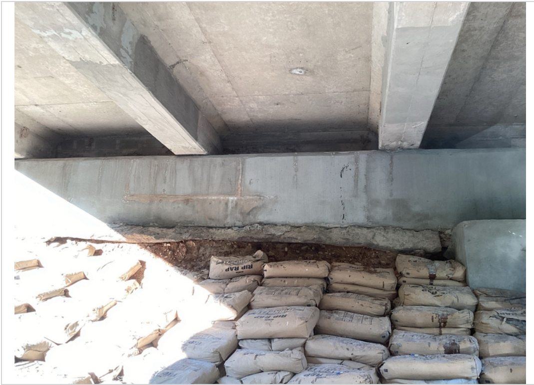
Abutment caps have been repaired with new concrete
