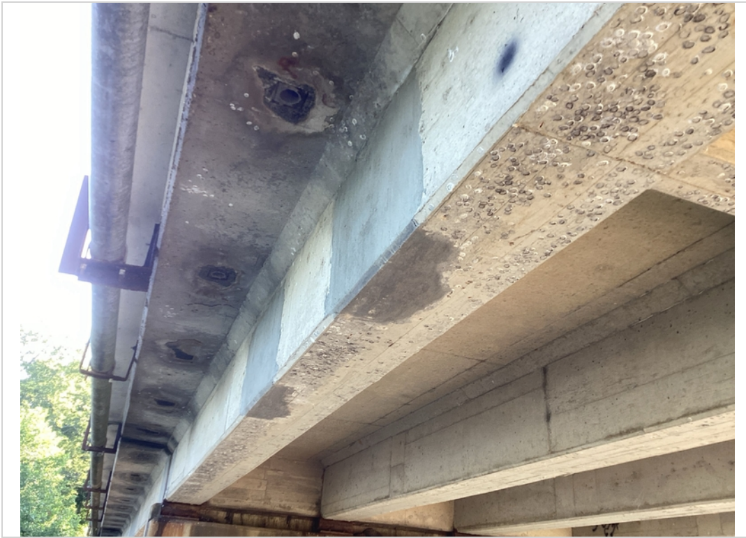
Crack repairs to beam "A" span #4
