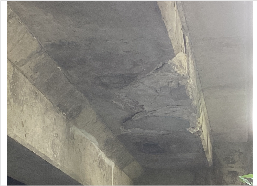
Span #9: In-place spalling right side overhang
