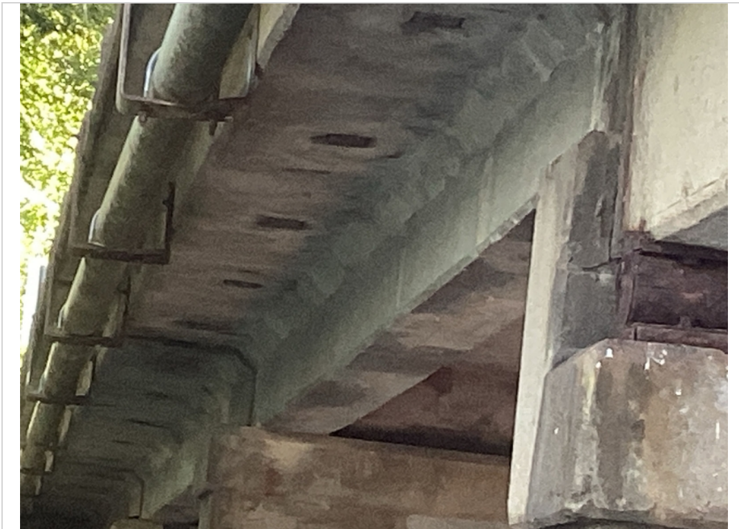
Crack repairs to beam "A" span #7
